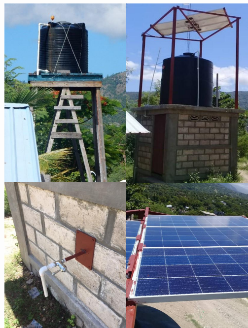
The old water tower (top left) and the new concrete water tower (top right) with solar panels and a 1,600 gallon tank. The spigot (bottom left) and solar panels (bottom right) are new features of the updated tower.
